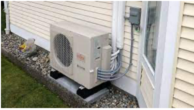
Outside unit needs 240V power and has the condensate drain
